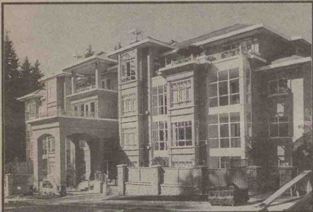
Raven Woods Phase 3 "The Legend" was part of a $13 million initiative that was built on the TSLEIL-WAUTUTH (First Nation Burrard Reserve)
