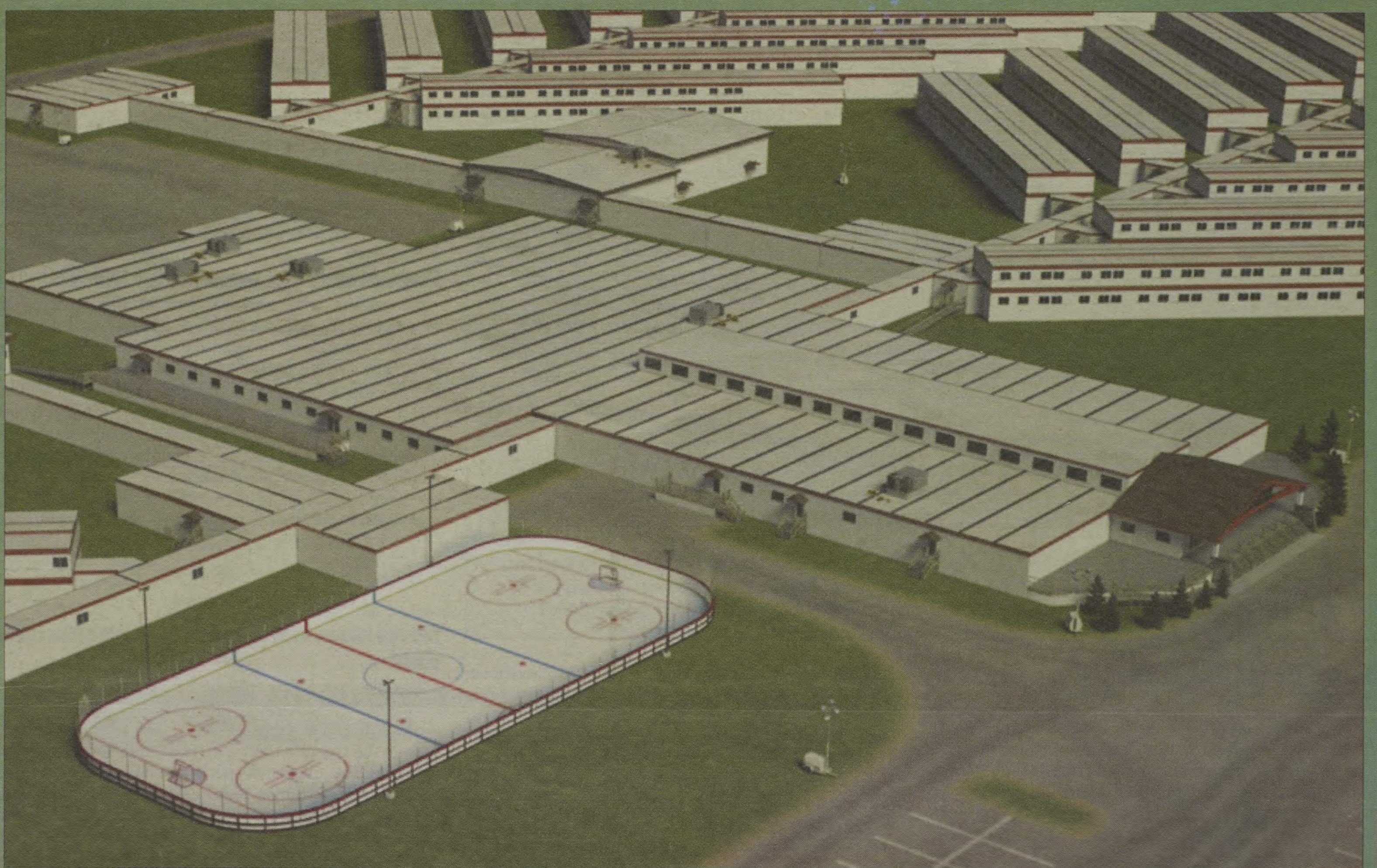
Artist rendition of the overall Touchwood Area camp that will house close to 2,600 workers for the Jansen mine.
